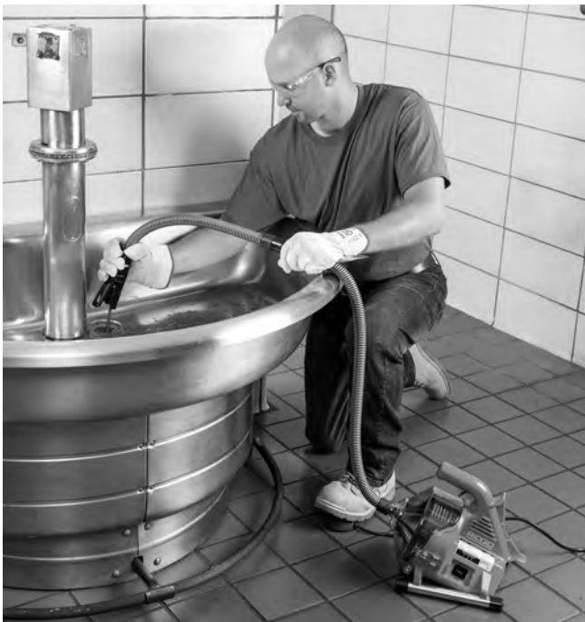
Figure 11 – Retrieving Cable
